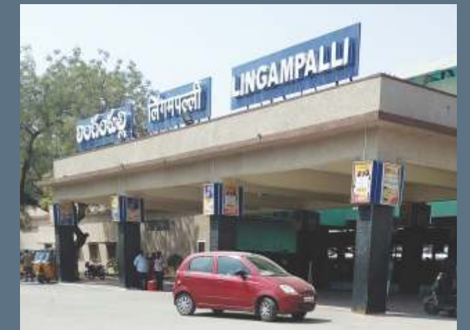
Lingampalli Railway Station
